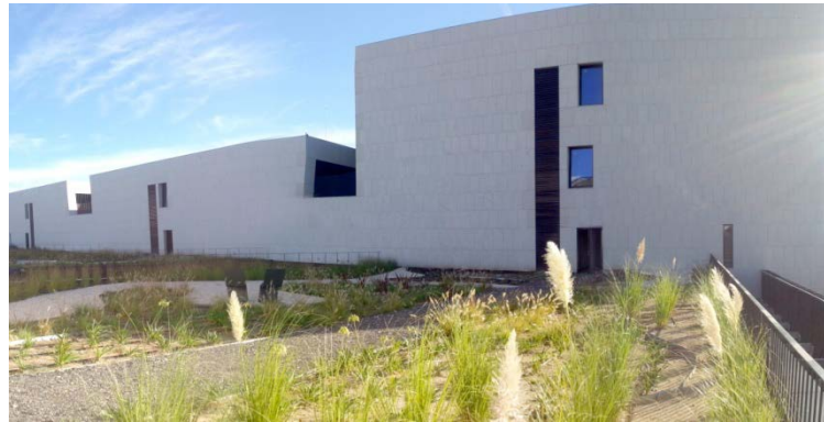
Hospital Collado Villalba, Madrid
