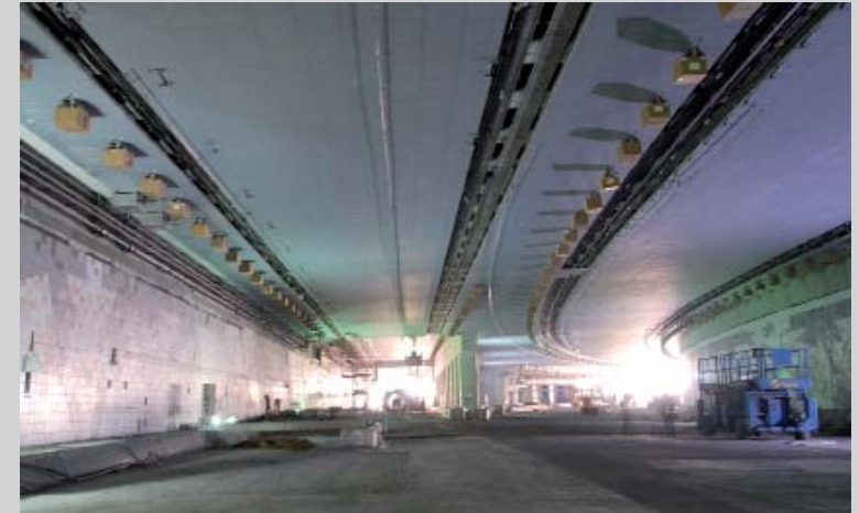
Túnel Al Salam Street, Abu Dhabi
