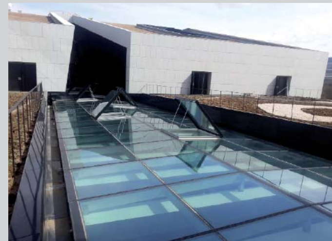
Hospital Collado Villalba, Madrid
