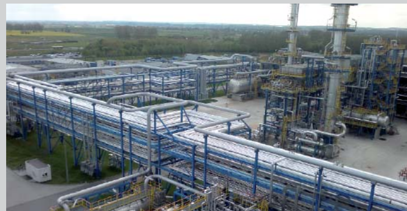
Mild-Hydrocracking Unit en Gdansk, Polonia
