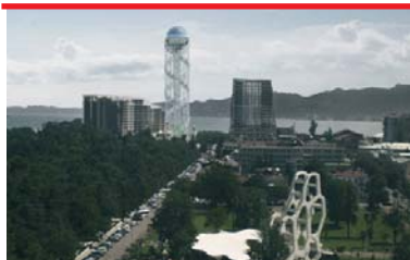
Alphabetic Tower in Georgia
