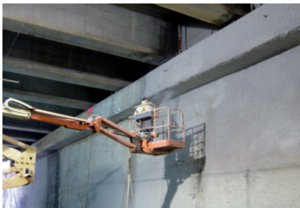
High Speed - AVE train Tunnel, Málaga (Spain)
