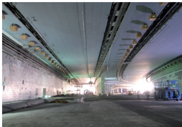
Al Salam Street Tunnel, Abu Dhabi (U.A.E.)
