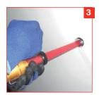
Once the cavity is filled in with **Tecfill®**, the operator will seal the holes made on the support work through the most suitable sealer (cement, plaster, mastic, etc)
