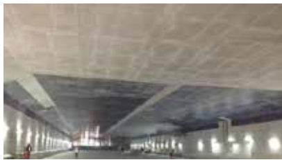
SINGAPORE SINGAPORE MARINA COASTAL TUNNEL E.XP. 482
