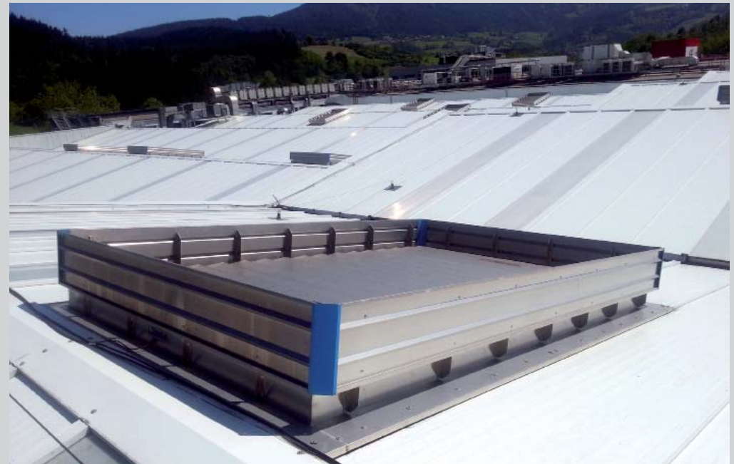
Eroski Logistic Center, Elorrio
