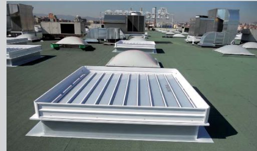
Alcampo Warehouse in Valdemoro, Madrid
