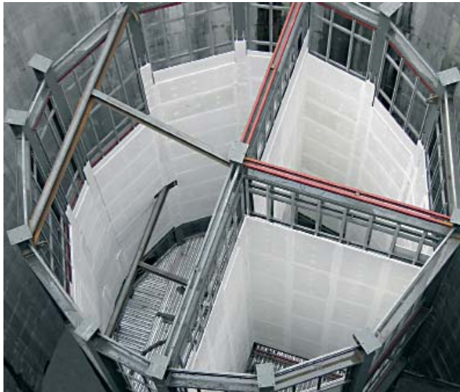
BY-PASS M-30 South, tunnel ventilation shafts, Madrid
