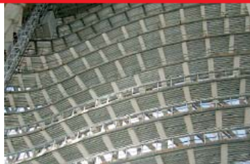
Expozaragoza 2008. Water Tower
