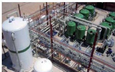
Unión Fenosa Combined Cycle Plant in Puerto Sagunto, Valencia
