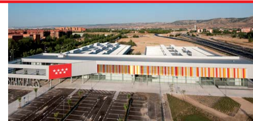
Sports Centre in Alcalá de Henares, Madrid
