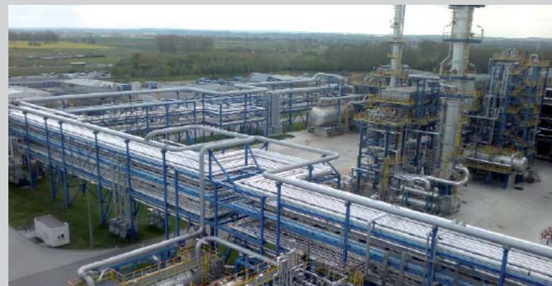
Mild-Hydrocracking Unit in Gdansk, Polonia
