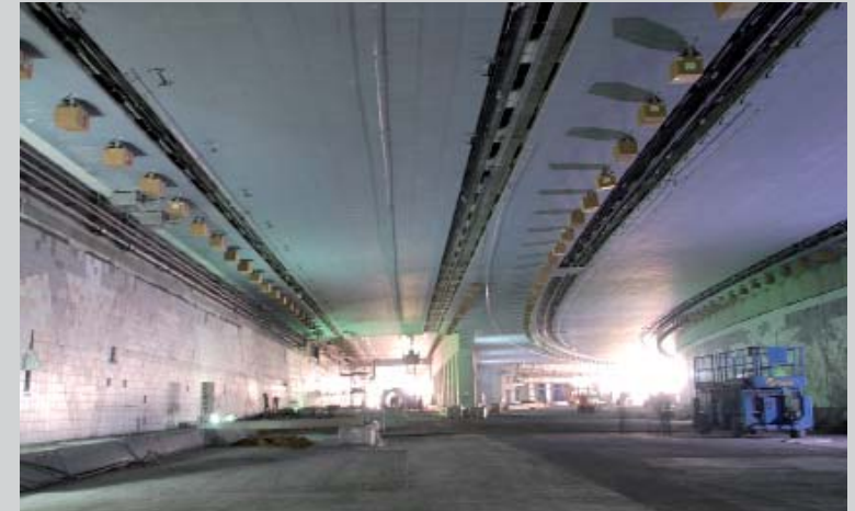
Al Salam Tunnel, Abu Dhabi
