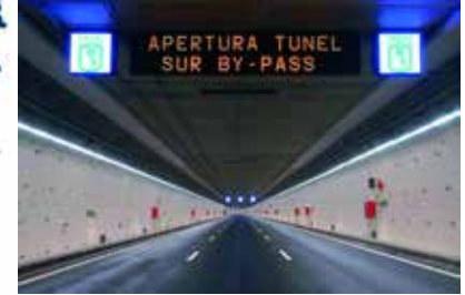
SPAIN MADRID M30 RING ROAD TUNNEL
