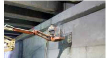
SPAIN MÁLAGA HIGH SPEED RAILWAY TUNNEL
