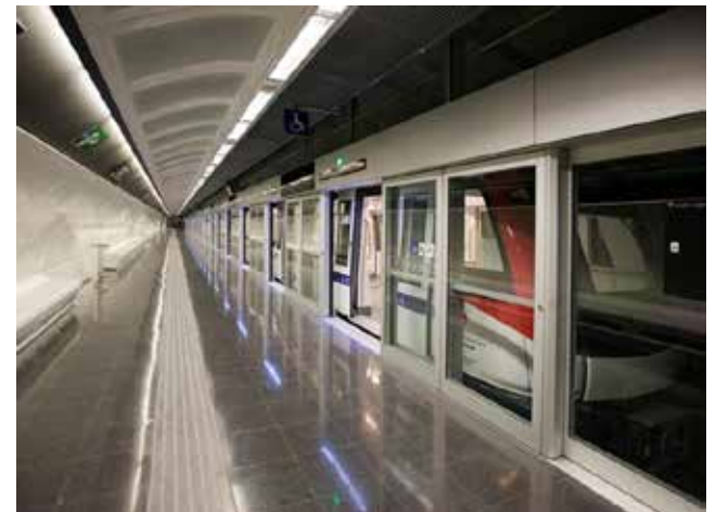
Line 9 Barcelona Underground, Spain
