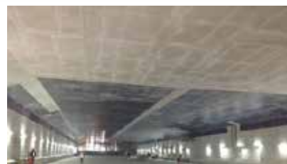
SINGAPORE SINGAPORE MARINA COASTAL E.XP. 482 TUNNEL
