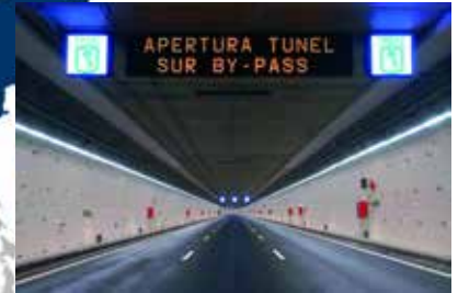
SPAIN MADRID M30 BYPASS TUNNEL
