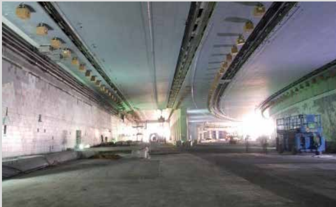
Al Salam Tunnel, Abu Dhabi
