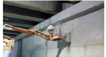
SPAIN MÁLAGA HIGH SPEED TRAIN TUNNEL- AVE
