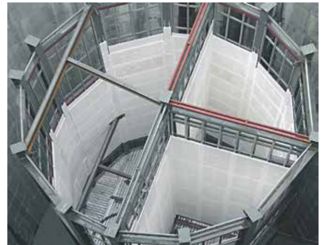
Ventilation shafts M-30 BY-PASS south tunnel, Madrid
