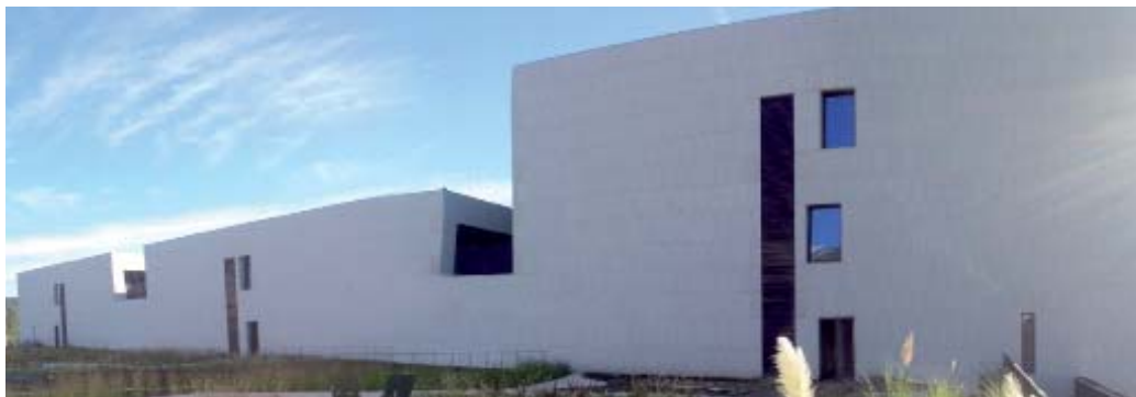
Collado Villalba Hospital, Madrid
