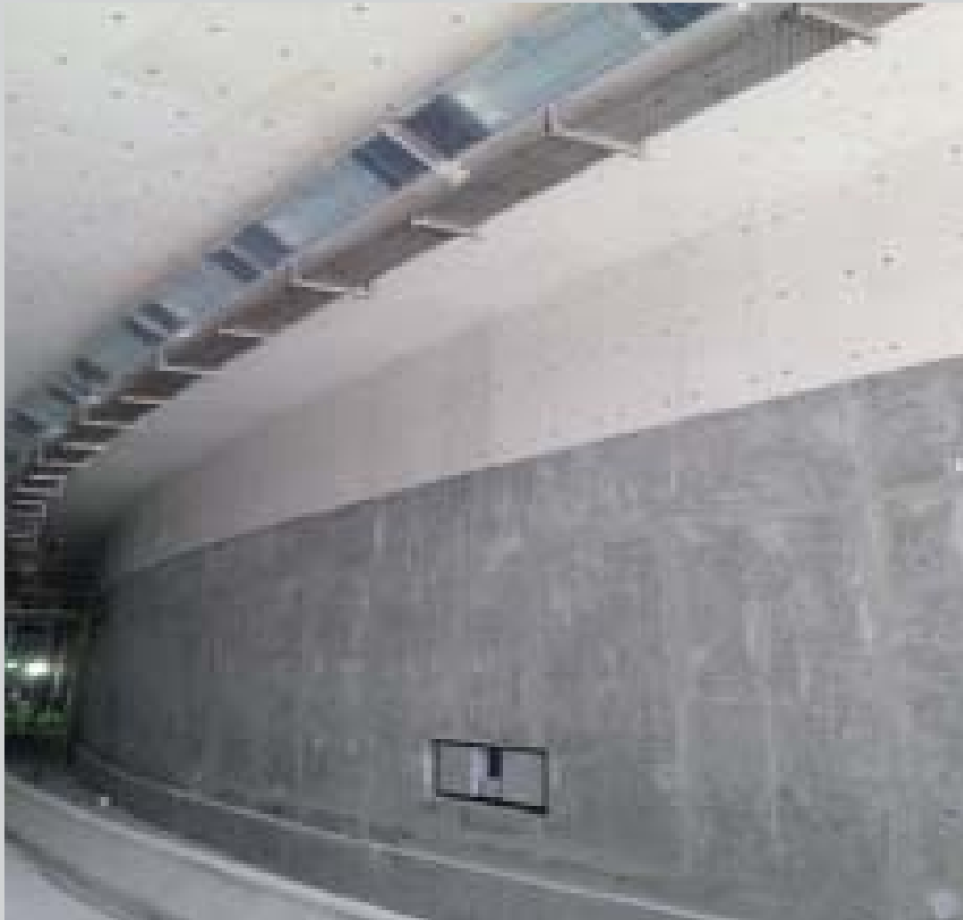
Al Ras Al Akhdar Tunnel - Baynoonah, Abu Dhabi.
